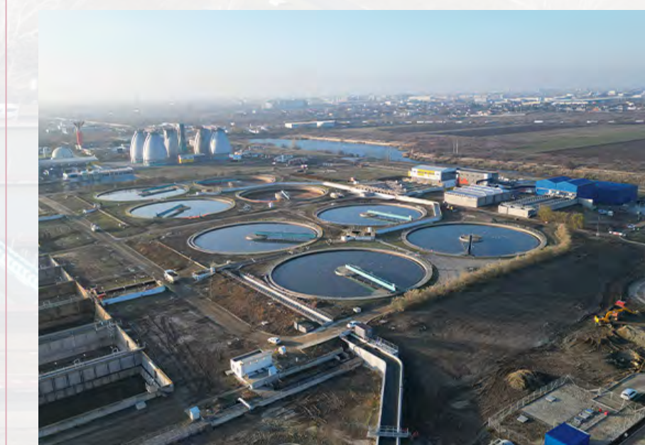
Decanters at the Glina WWTP in Bucharest, Romania
