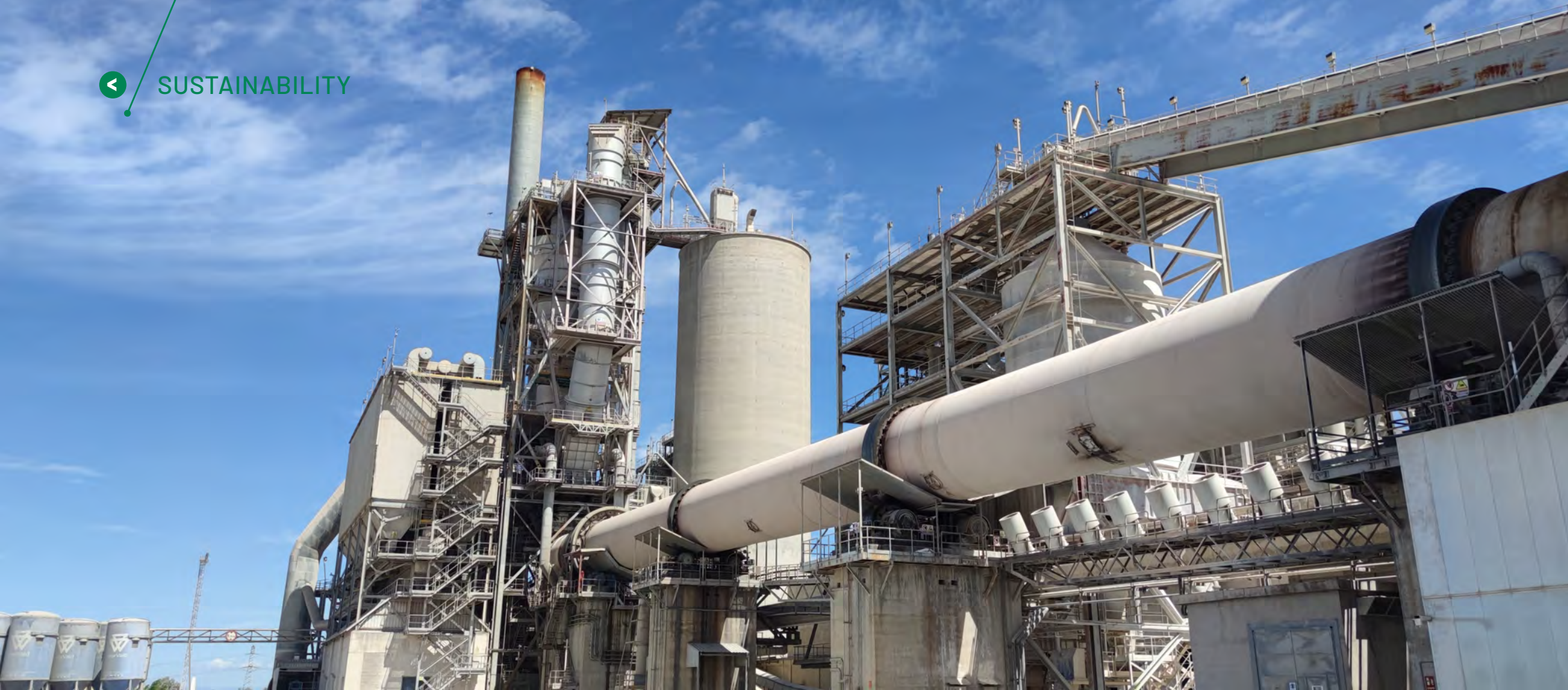
Cementos Portland Valderrivas' plant in Morata de Tajuña, Madrid.
